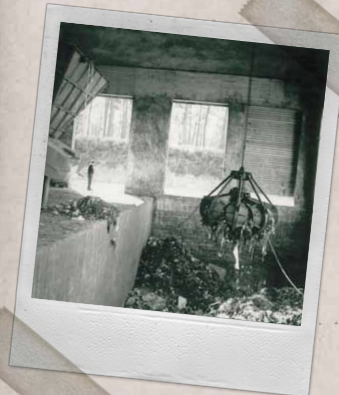
Fossa de descarga da Antiga Central de Compostagem Discharge tank of the former Composting Plant.
