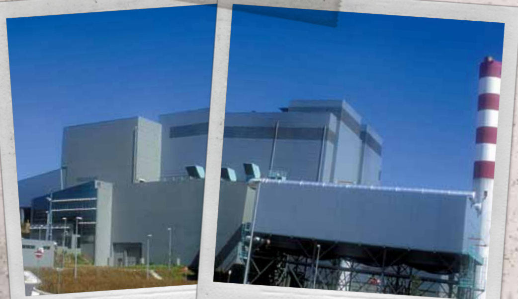
External view of the Energy Recovery Plant
